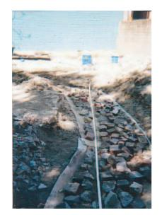
Creekbeds are placed during site excavation, filled with sand and rubble, and packed down to avoid subsidence.
